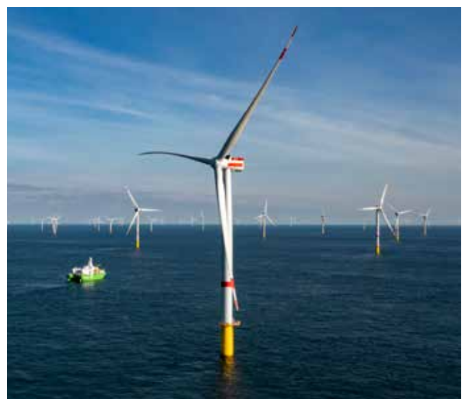
Figure 5. Example of a Monopile Foundation Type at Ocean Winds' Seamade Wind Farm in Belgium.
