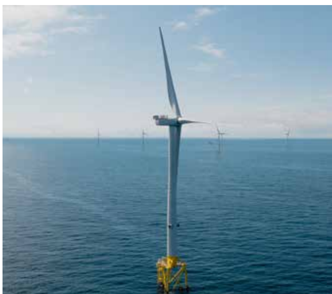
Figure 4. Example of Jacket Foundation Type at Ocean Winds' Moray East Wind Farm in Scotland.
